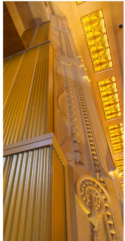
Turning the site of an abandoned auto factory into a glamorous casino is no easy task. Pilkington Profilit™ low-iron, wave channel glass with TGP ProColor® translucent metallic gold coating helped the design team for the Hollywood Casino in Columbus, Ohio, achieve this goal by capturing the golden age of Hollywood from the outside in.
