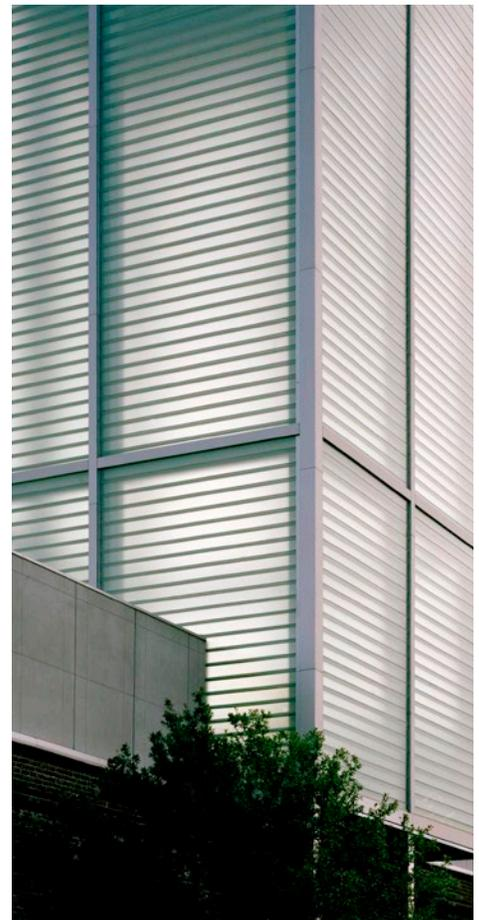
Grafted onto the 19th-century brick remains of the Savannah College of Art and Design (SCAD) Museum of Art is an 86-foot tall, semi-transparent channel glass tower. It is the first application to use hurricane-rated channel glass in a horizontal, dual-glazed configuration without additional support.
