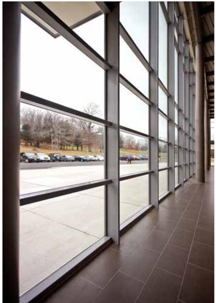
The firm chose SteelBuilt Curtainwall Infinity™ SSG System from Technical Glass Products, Snoqualmie, Washington. The steel-based curtain wall framing system is typically three times stronger than aluminum assemblies of the same profile dimension, allowing for reduced frame dimensions and greater free spans of glazing, both of which are necessary for increasing daylight and views.
