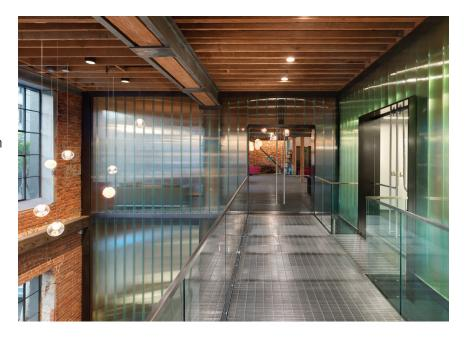
For the glazing throughout the lobby, the architects chose Pilkington Profilit<sup>™</sup> channel glass from Technical Glass Products (TGP). The linear, "U"shaped, cast-glass channels are self-supporting and mounted in a custom framing system fabricated by Chris French Metals and designed by MacCracken Architects.
