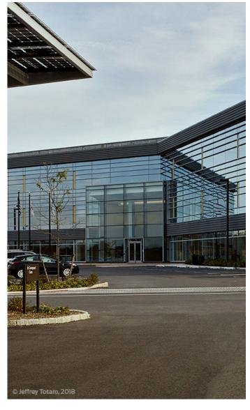
With no exterior caps and minimal back mullions, the resulting system allows for uninterrupted exterior sightlines and the desired smooth glass-to-glass, butt-glazed appearance. The steel framing also supports exterior-mounted sunshades. This lessens direct solar transmittance through the glass and helps cut down on glare when looking out through the wall to the exterior.
